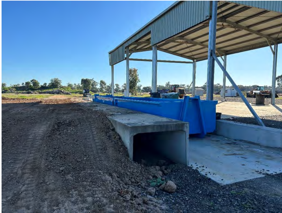
Extra earthworks to support blue bin deposits
